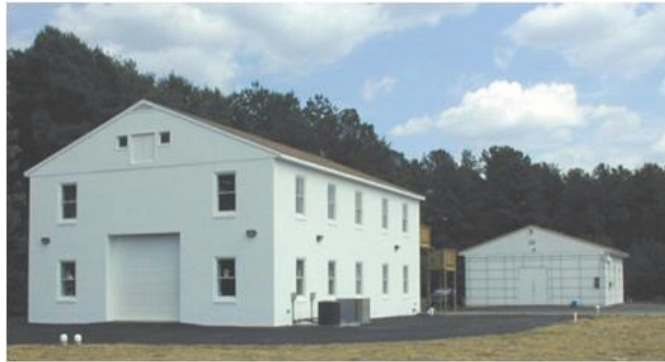
Figure 8: MOATS HPM test facility
