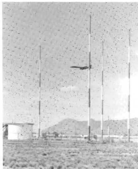
ATHAMAS II, resistively-loaded wire-cage cone, 40m tall. A B1-B is landing in background.
