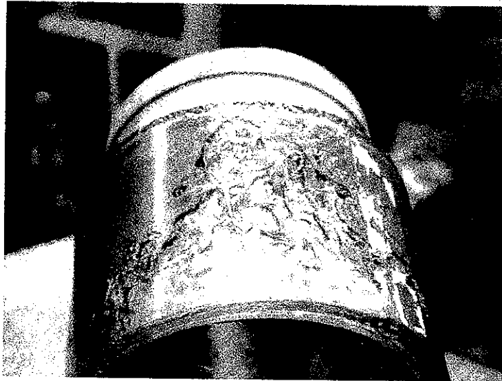
Figure 3-15. Bubbles in Epoxy Caused by Run Away Exotherm
