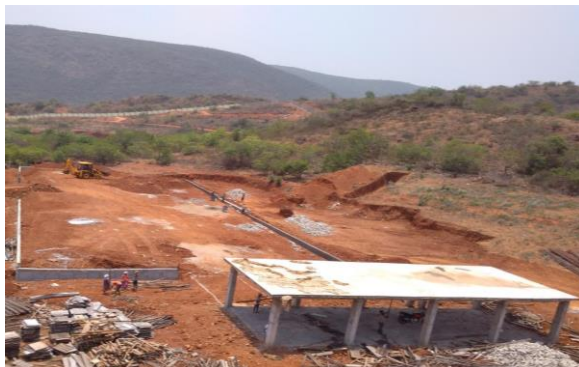
Figure 11. RS105 test facility- Construction Progress.
