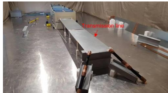
Figure 12. Verification of RS105 Generator - Metal plate & bank of resistors
